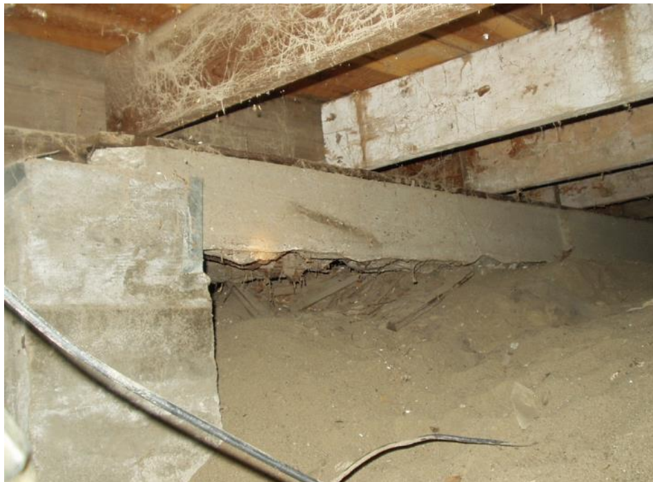
Figure 4: Undermined Grade Beam
